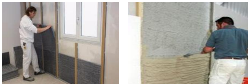
Figur 5. Aerogels application as a thermal insulation for inner wall,
